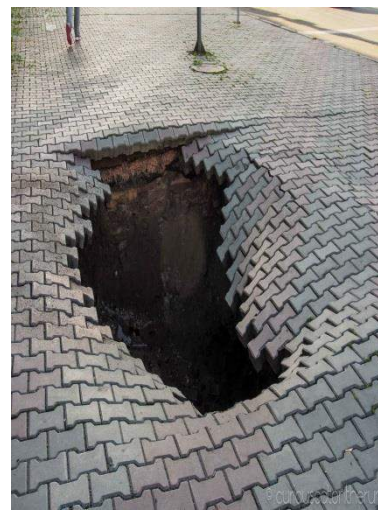
Landed on pavement from a 100 feet vertical fall
