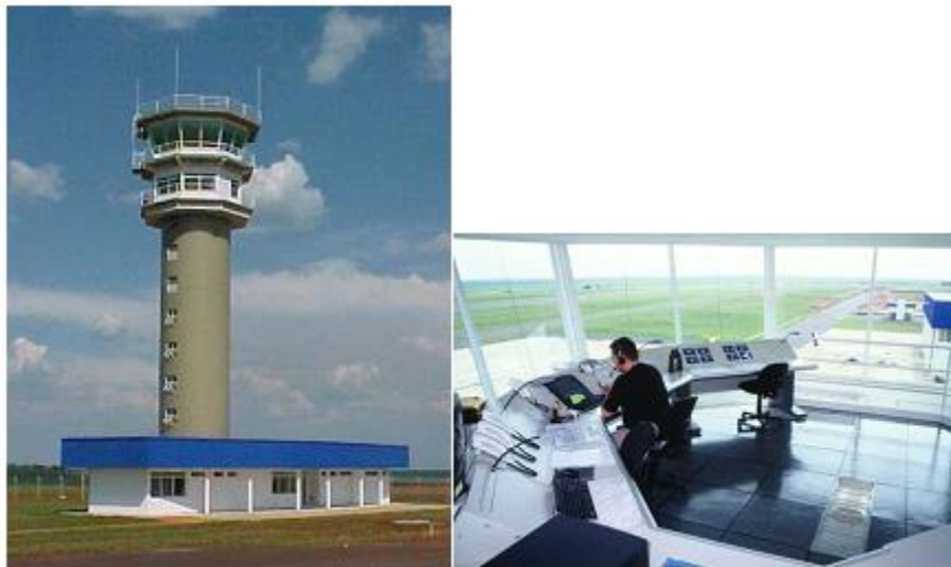
Figure 3: AeroMACS Base Radio installation in the Embraer Command Tower.
